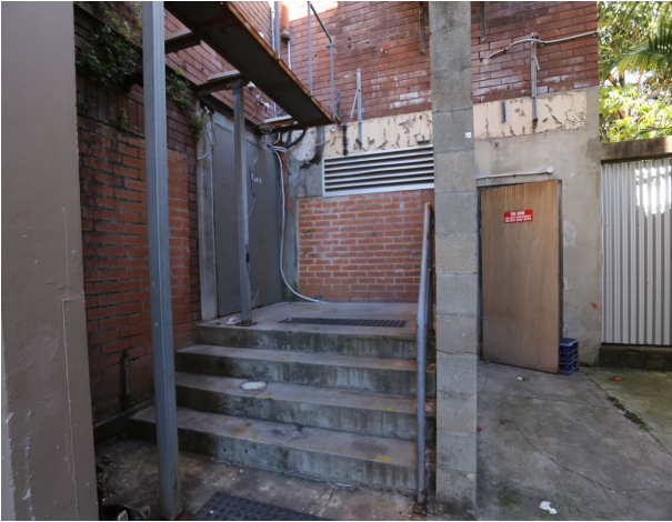
Figure 152 – Views of the western façade from Hourigan Lane.
