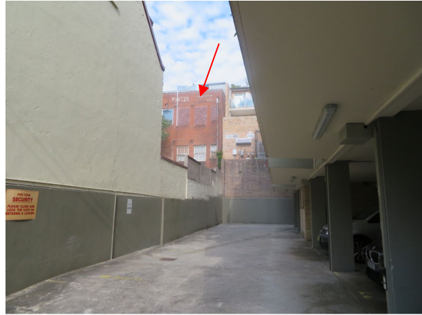
Figure 153 – Views from Brougham Street of the top corner of the western façade (indicated).
