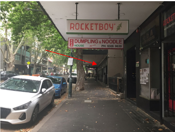
Figure 150 – View south on the western side of Victoria Street. The ground floor of the subject site is indicated.
